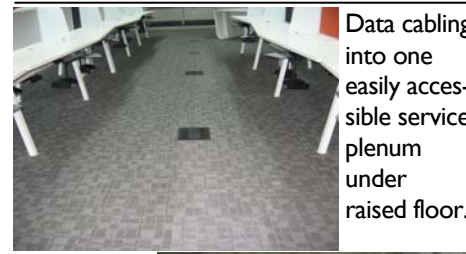
These raised floor systems are particularly appropriate for office buildings
